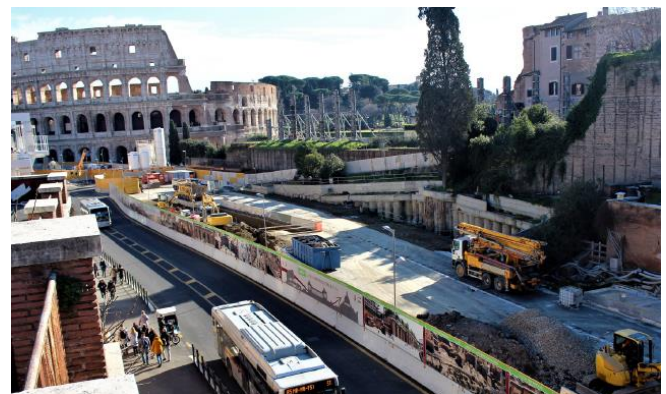
Figure 2 aerial view of the Metro C – Fori Imperiali job-site.
